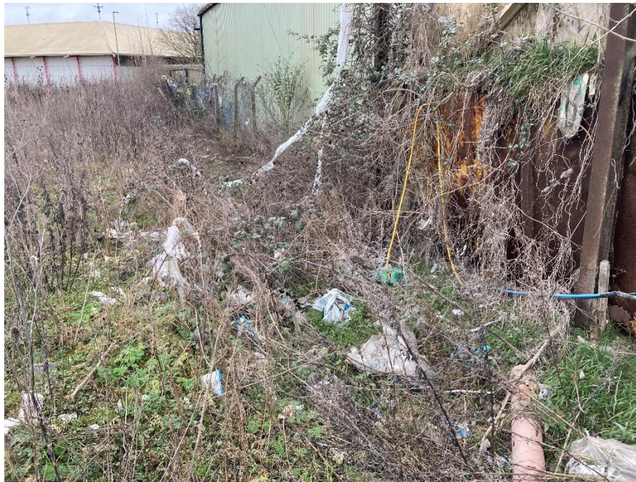
Inert waste located on the east boundary of Site.
